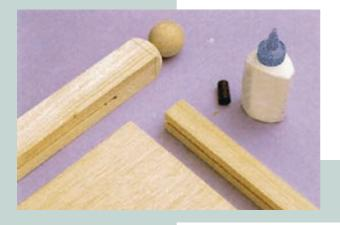
Joining and gluing of the flower pot is then performed in two steps. First, join the frame strips and side elements together while adding glue (waterproof). The plywood must protrude laterally by 10 mm. This protruding section is then stuck into the post grooves which have been coated with glue. The gluing surface of the joint is sufficiently large to permit the frame strips to make flush contact.
