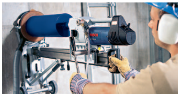
Wet drilling with a system: Bosch Diamond Drill GDB 2500 WE, diamond core cutters, Drill Stand S 500 A, dust extraction device and all-purpose vacuum cleaner.
