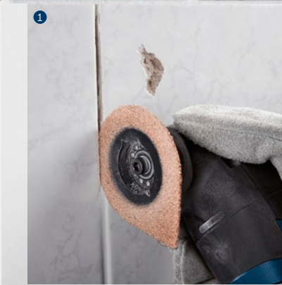
Routing joints on wall and floor tiles.
