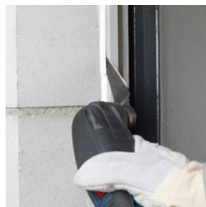
Cutting soft expansion joints.
