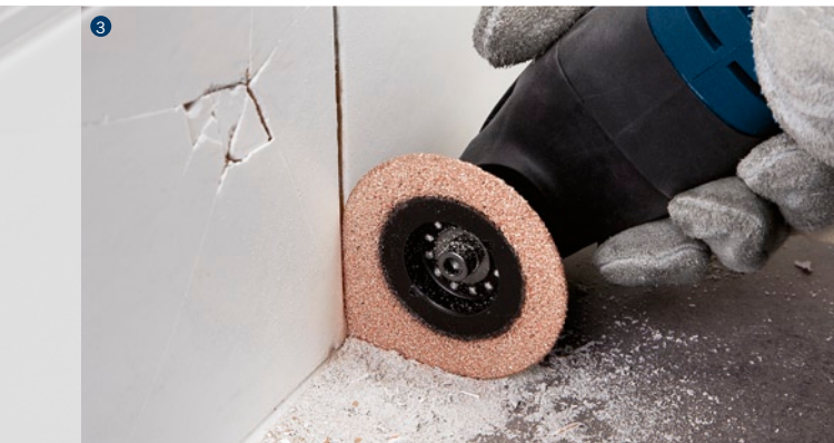
Routing joints right into 90 degree corners.
