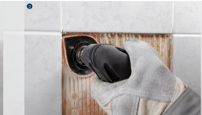
Removing mortar or tile adhesive – even right into corners.
