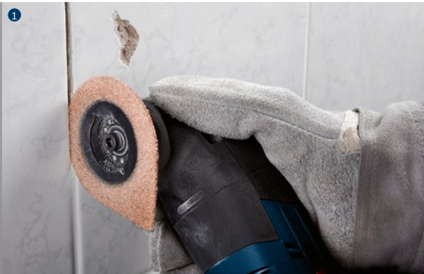
Routing joints on wall and floor tiles.
