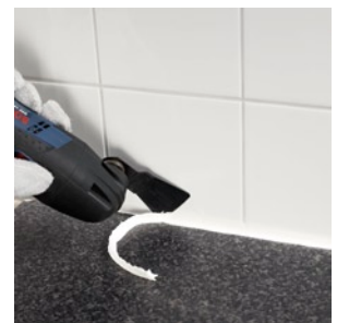
Removing old silicone joints.
