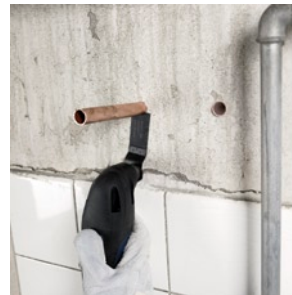
Flush cutting of a protruding copper pipe.
