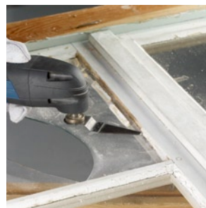
Cutting window putty (sealing compound).
