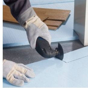
Cutting sound dampening panels to size cleanly and efficiently.
