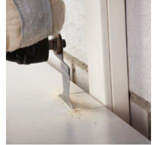
Precise plunge cuts in laminated panels, e.g. recess for a shelf board.
